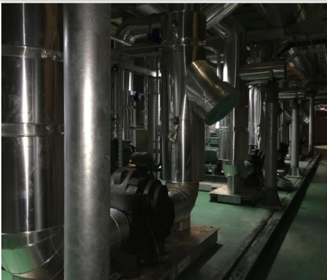
Compressor of petrochemical factory
